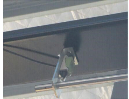
Picture 10 ( up limit switch connection)
